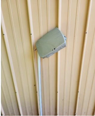
Outside fiber enclosure (NID) Above: Damaged from improper removal. Below: Proper installation.
