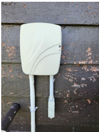
Outside fiber enclosure (NID) Above: Damaged from improper removal. Below: Proper installation.
